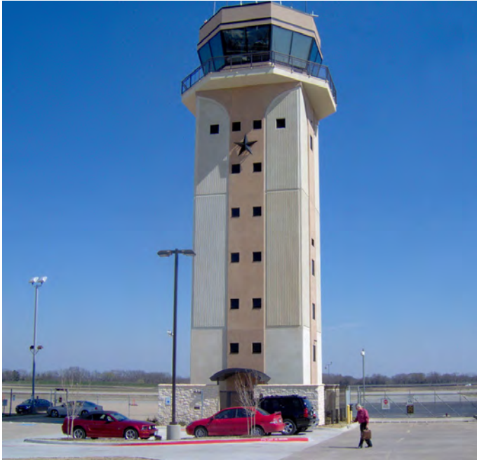
The new McKinney, Texas, ATCT that was commissioned on Feb. 16, 2011.
