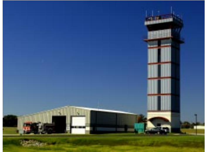
Donaldson Center's New Air Traffic Control Tower
